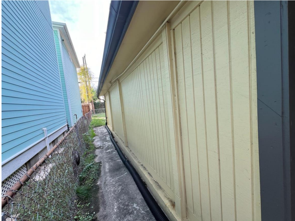
SOUTH ELEVATION OF SIDE WALL NOT COVERED BY CARPORT
