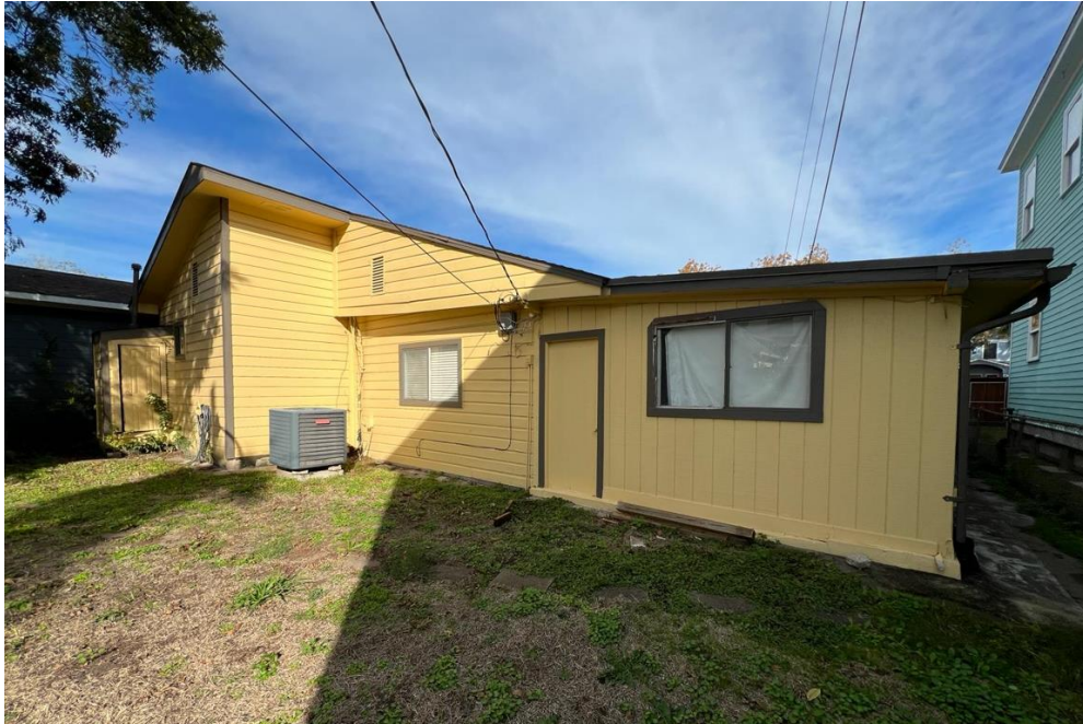
OBLIQUE VIEW OF WEST (REAR) ELEVATION
